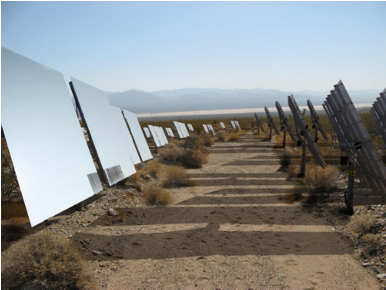
The Ivanpah valley solar power plant, being built by BrightSource (Image: BrightSource)
